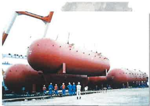
● Vessel(槽)水切工事
